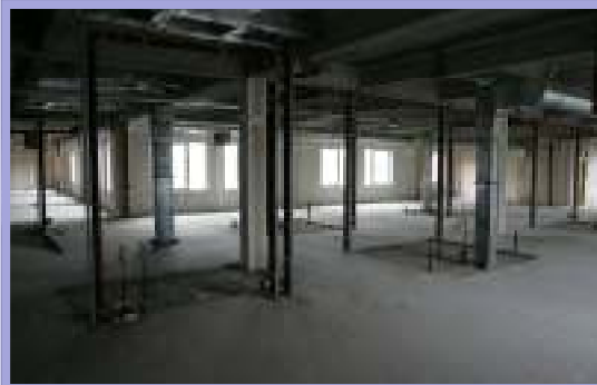
Empty shell space on level 4 of Golden Jubilee National Hospital
