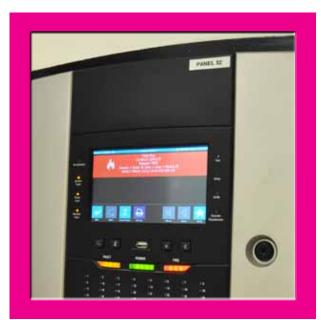
An intermittent alarm will sound in compartments adjacent to where the continuous fire alarm is sounding. The intermittent alarm is a warning alarm that allows staff to become prepared for a possible evacuation from their compartment, should a continuous alarm be sounded.
