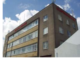
The Dental Directorate Clutha House 120 Cornwall Street South Kinning Park, Glasgow
